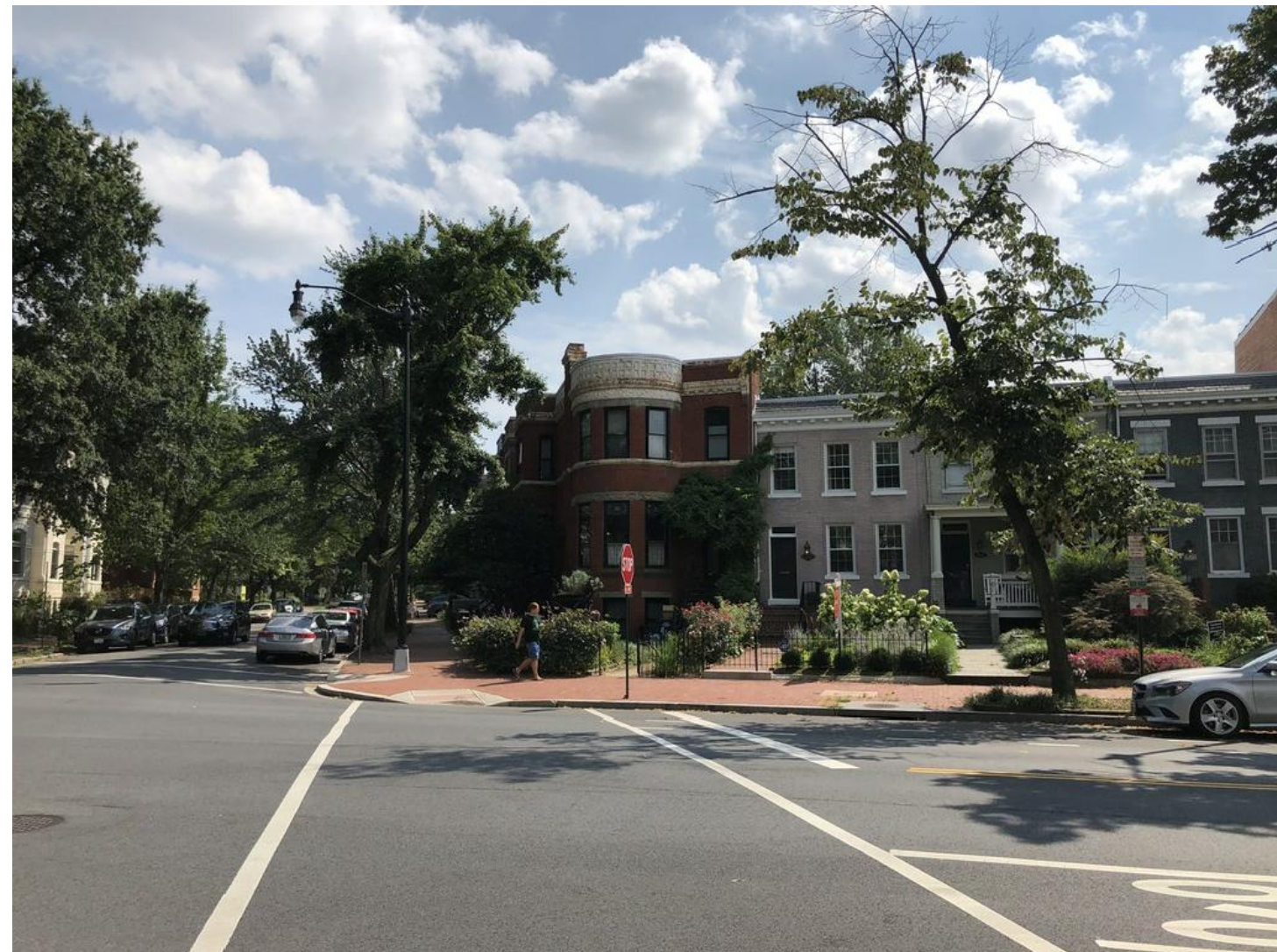
PHOTO A NO ROOFTOP ELEMENTS ARE VISIBLE.
